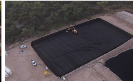
4. Geomembrane installation
