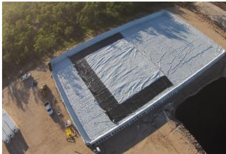
5. Primary liner installation
