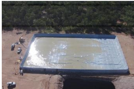
6. Secondary liner installation
