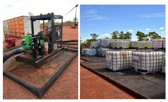
Figure 14: Example of spill mats used to contain potential contaminants
