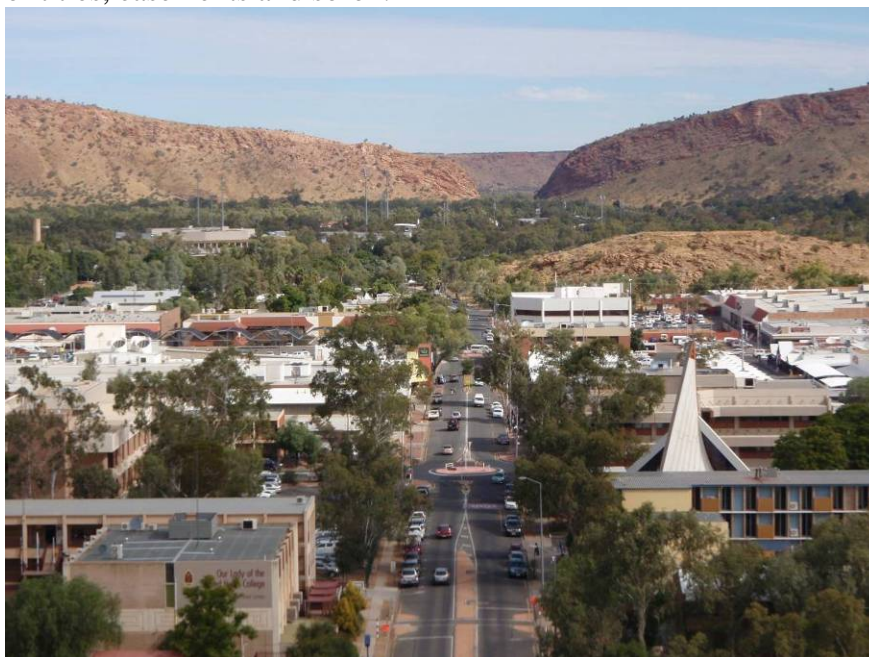
View of Alice Springs looking south towards Heavitree Gap 2011
