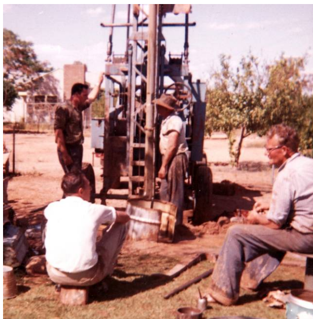
Sandy Cole (of Gorey & Cole Water Drillers) and Allan Burrows, seated, & others drilling domestic water bore into Town Basin on East Side 1963
