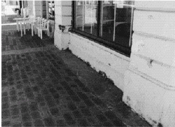
Damage to shops in the main street of Pingelly (November 1998) due to rising damp and fretting of brick walls.
