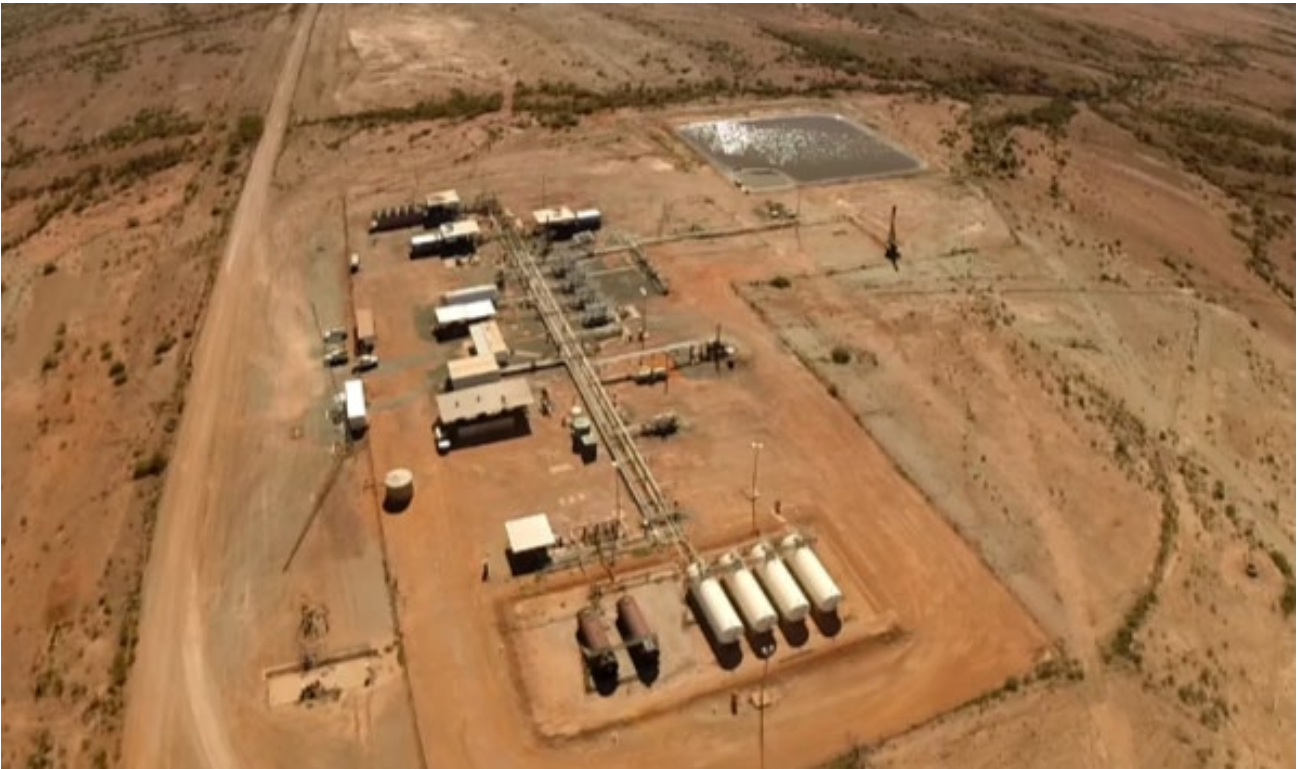
Figure 3-5 Aerial view of Eastern Satellite Station
