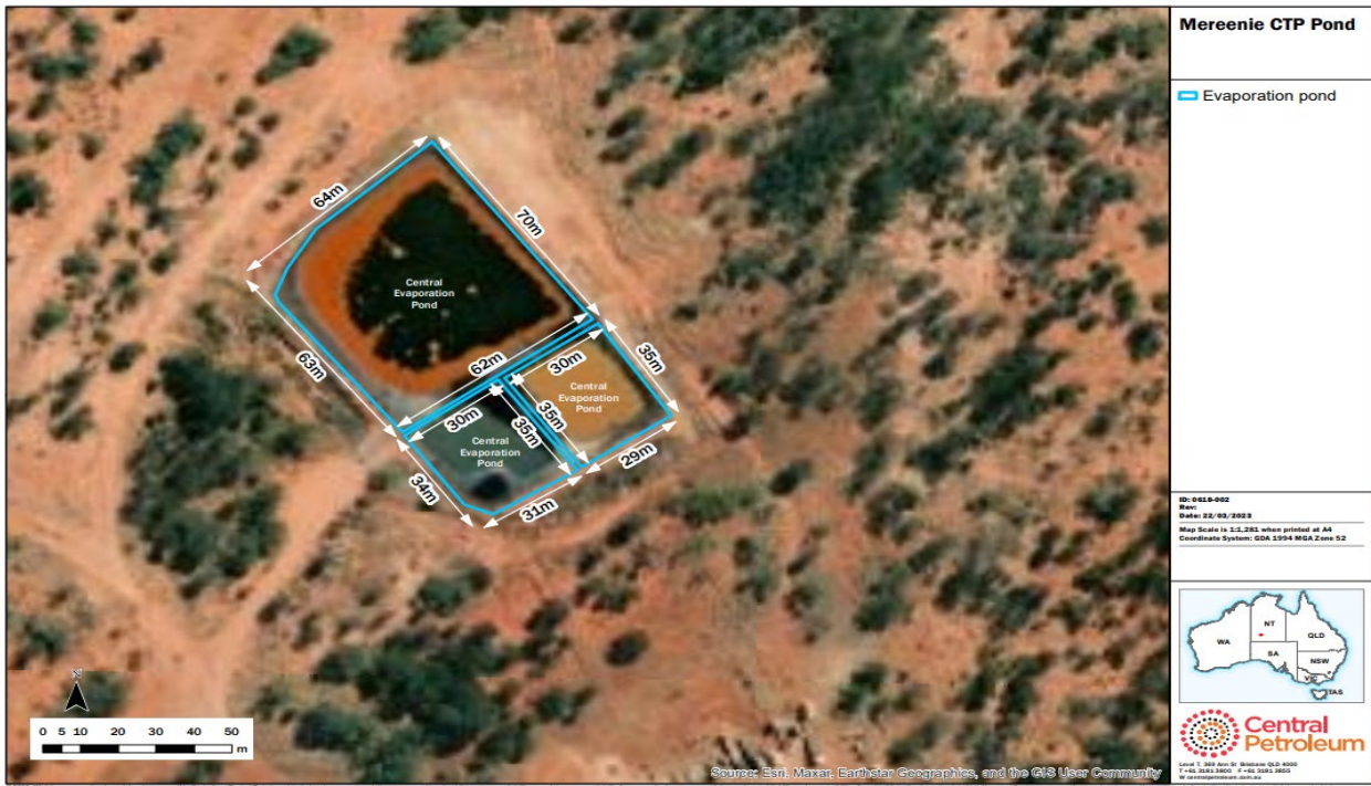
Figure 3-8: CTP Wastewater solar evaporation ponds
