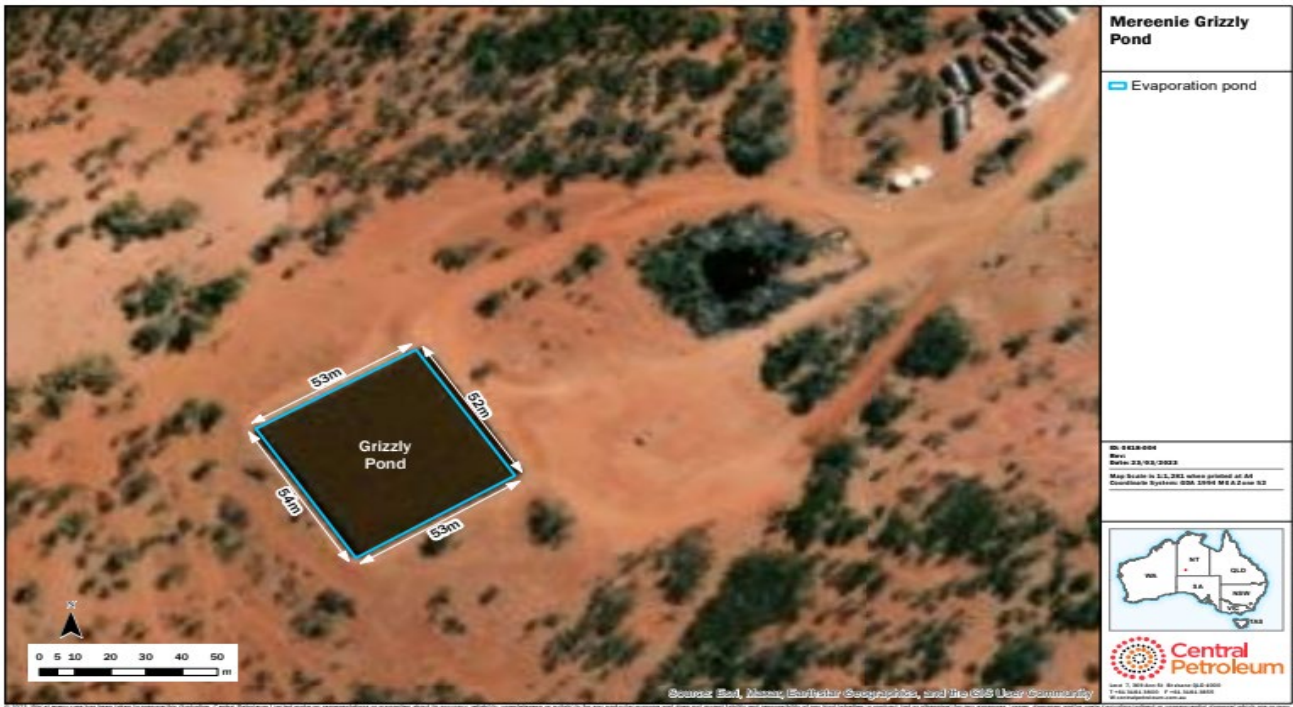
Figure 3-10: Grizzly pond Wastewater solar evaporation pond
