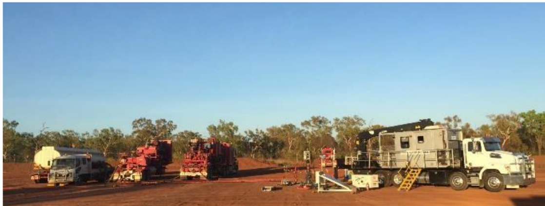
Figure 1: Image of equipment utilised to perform a DFIT, including wireline unit, water truck and pump trucks.
